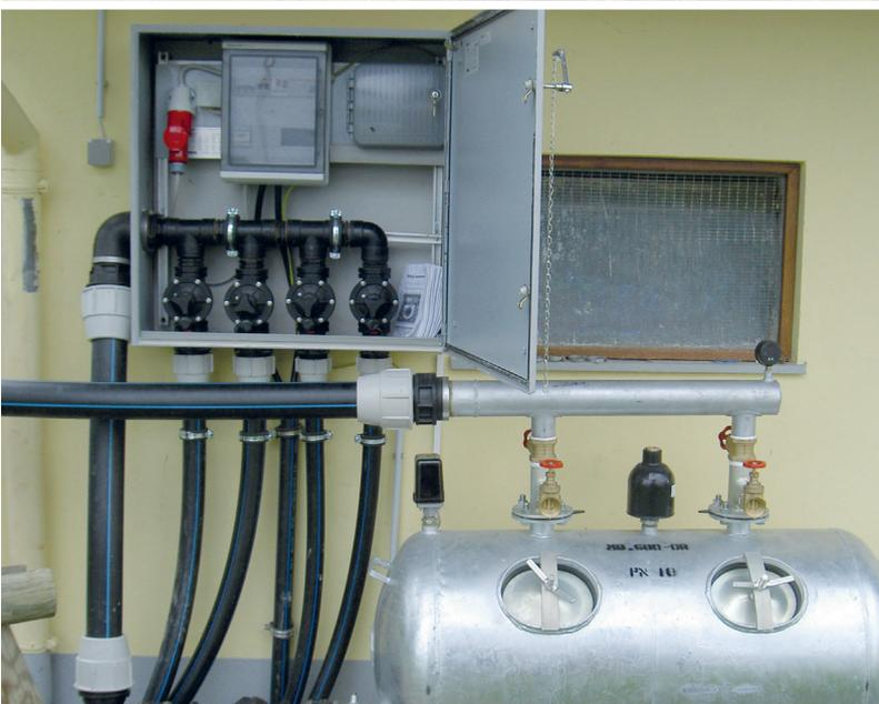
Automatic controls with manual filter system
